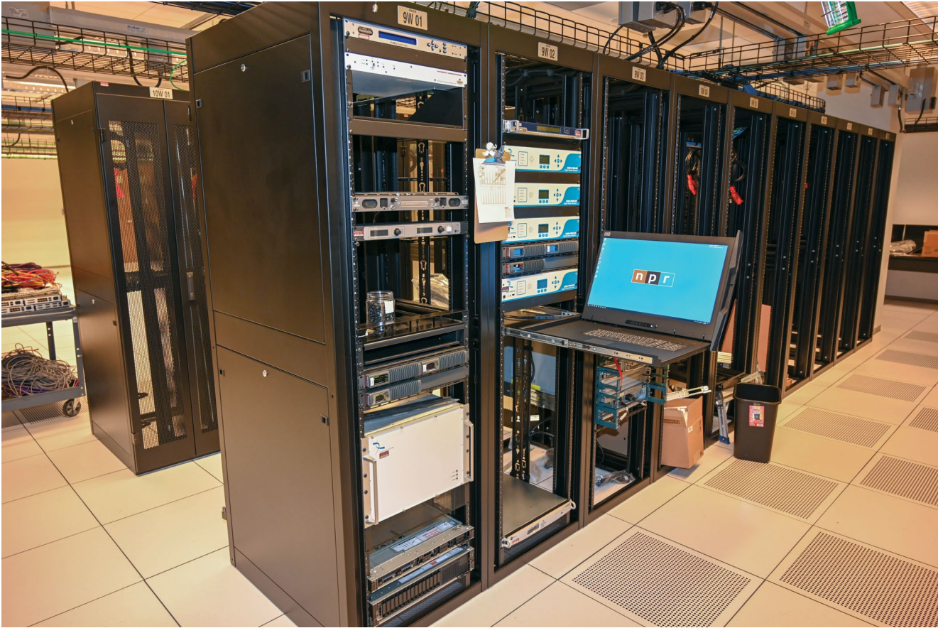
Fig. 1: Initial development environment equipment racks are shown installed. The first rack on left has, from the top, a system master clock, clock distribution amplifier, Wohler monitor amplifier, Axia selector panel, Axia AES audio node and ATX encoding equipment below.
