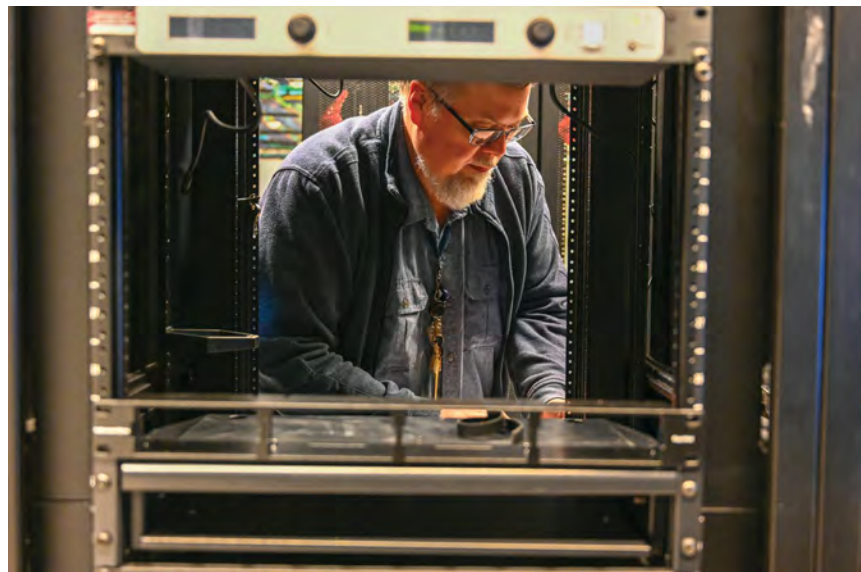
Fig. 3: NPR Senior Distribution Systems Architect Doug Bevington installs cable management for system racks.
